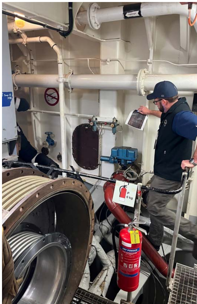
MXAK Inspector verifying valve closure at physical location.
